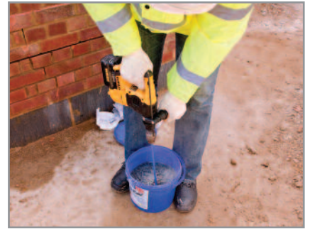
3. Stir thoroughly using a power-driven paddle mixer. Do not attempt to mix by hand as this will result in inadequate mixing
